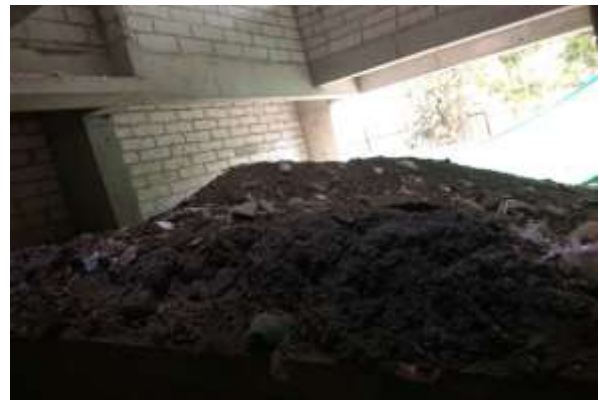
Fig. wastage of cement, sand and blocks
