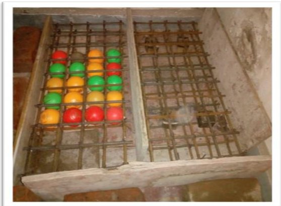
Figure 4: Formwork of slabs
