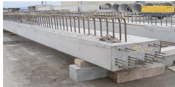
Fig.: Prestressed Beam
