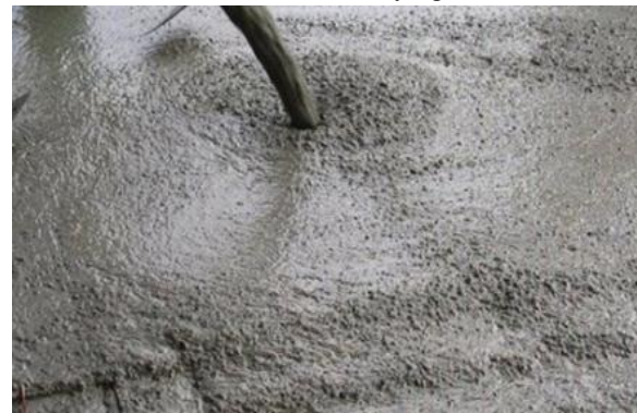
Fig.: Self compacting concrete
