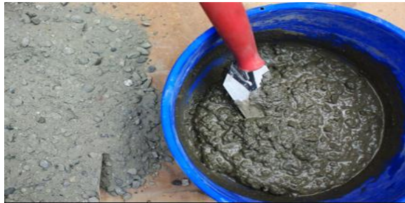
Fig.: Mixing of concrete
