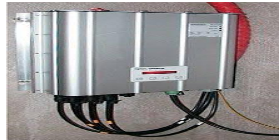
Fig. 2.2: Inverter for grid connected PV
