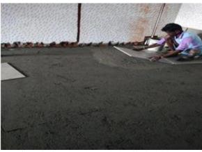
The floor is first leveled and the tile is laid. Glazed vitrified tile (2' x 2') is used for floor. The thickness of tile is 90mm for both floor and wall. The minium rate of tile starts from Rs.25. After laying the tiles the floor care gypsum powder is mixed with the water and poured over the tiles.
