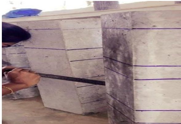
Figure 1. Marking of column
