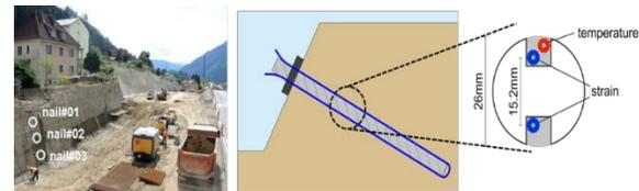
Figure 10. Fibre optic equipped soil nails at a construction site with three sensing nails (left) and their cable layout (right)
