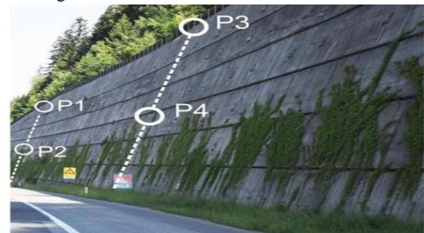
Figure 2. Prism positions for the geodetic monitoring of a retaining wall
