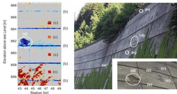
Figure 5. Automatically detected significant deviations from the linear regression lines (left), images of the retaining wall with prism positions P1 and P2 and local damage d (right)
