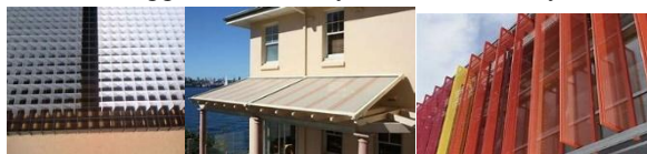
Eggcrate rotating horizontal louvers, External frames with movable awnings, rotating vertical fins
