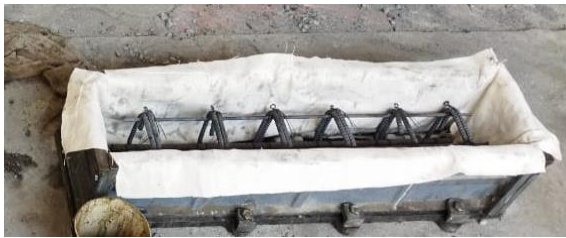
Fig 5 Reinforcement of lightweight concrete using liner
