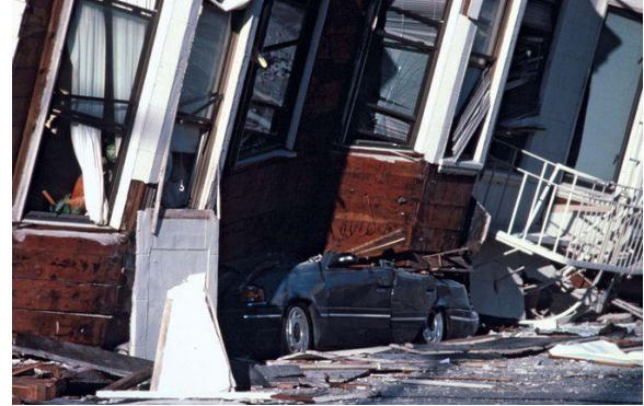
Loma Prieta earthquake of 1989: soil liquefaction An automobile crushed under the remains of an apartment building in the Marina District, San Francisco, California. The first and second floors are no longer visible because of structural failure and sinking due to liquefaction during the Loma Prieta earthquake in 1989.
