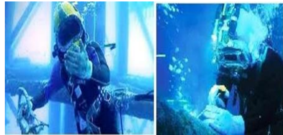
Welder/ Diver Performing Underwater Inspection by NDT Method
