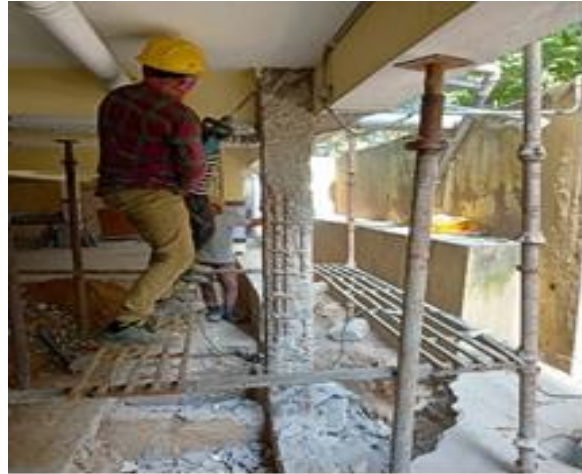
Figure-5 : Chipping of concrete
