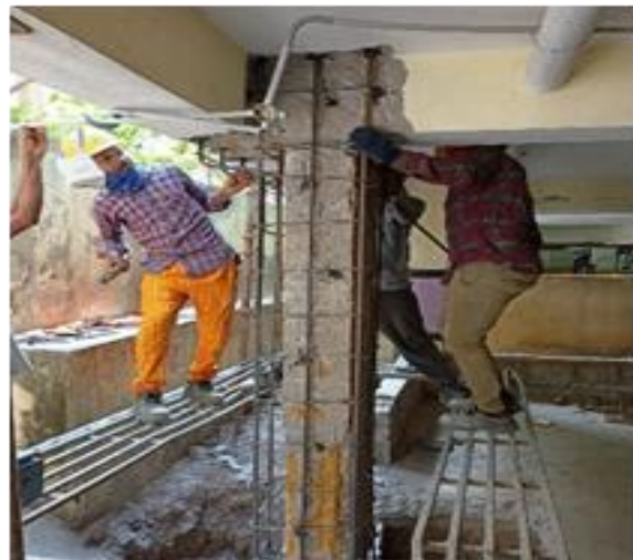
Figure-6 : Fixing of additional reinforcement
