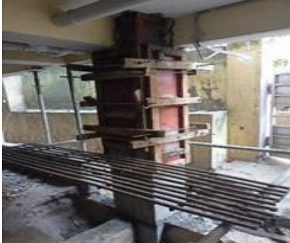
Figure-7: Shuttering
