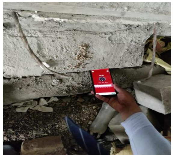
Figure 2. Pictures showing measurement of sound insulation of the walls.
