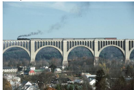
Fig 1 Deck Arch Bridge
