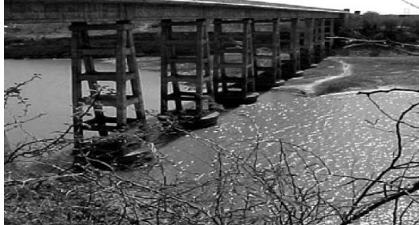
Fig.5 The Rudramata Bridge
