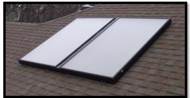
Figure 5 Flat plate solar collector
