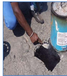
Fig. 10 Poring TGP and leveling
