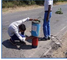
Fig. 4 Shredded plastic Fig. 5 Heating at site Fig. 6 String while heating Fig. 7 Cleaning pothole.
