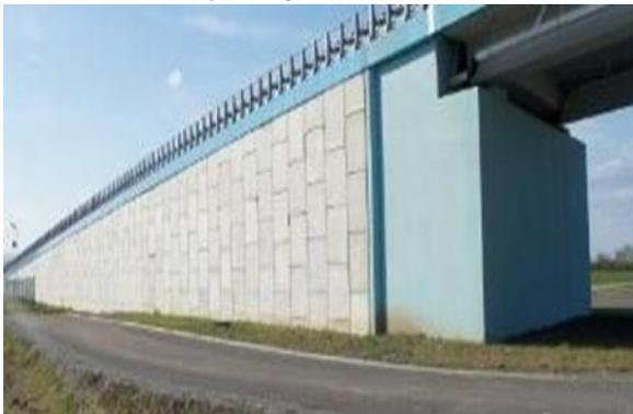
Fig. 1.2: Reinforced soil retaining wall constructed for highway structures
