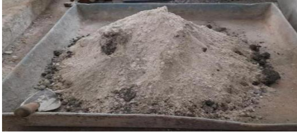
Fig 5. Mixing the sand and cement
