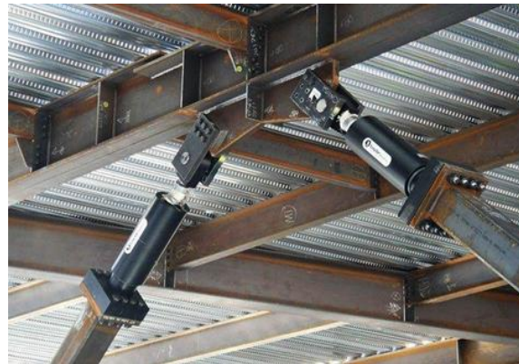
FIGURE 2: Incorporation of dampers
