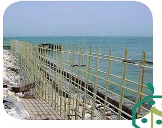
FIG.2 SEA WALL CONSTRUCTION
