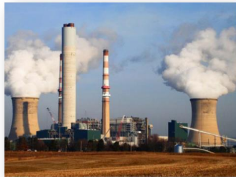
Figure 1.1. Industrial RC chimney
