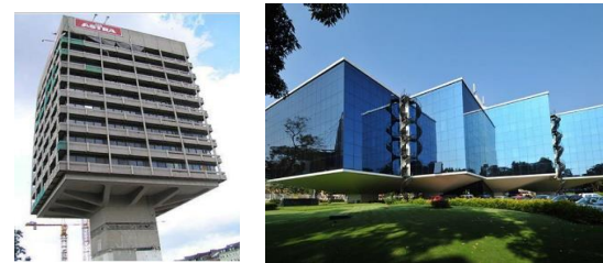
Astra house building Hamburg , Germany L&T Headquarters building Manapakkam ,Chennai
