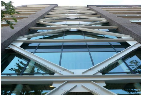
Figure 1.1 : X-bracing (cross bracing) system
