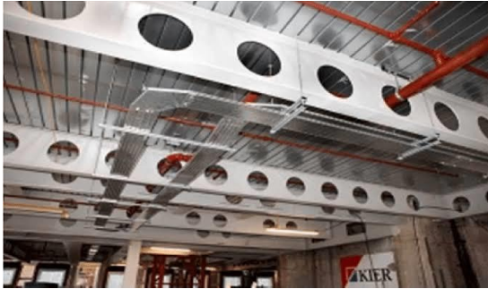
FIG-1.1 CFS SECTION WITH PERFORATION
