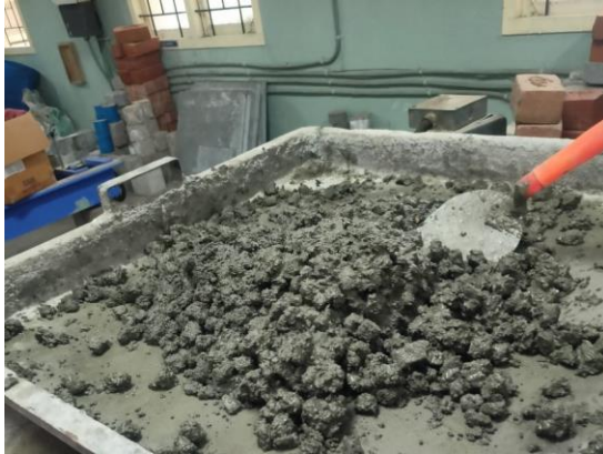
Fig 5.5 Mixing of concrete
