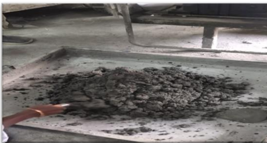
Fig 5.1 Mixing of Conventional Concrete
