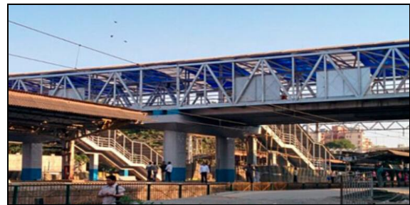
Fig 1 Foot over Bridge
