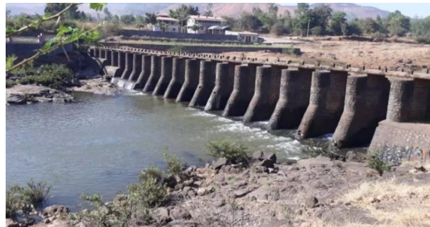
Fig 1 Bridge Cum Bandhara
