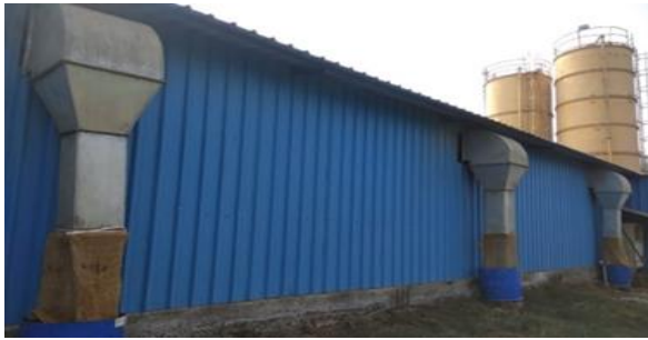
Fig 11 Controlling cement dust emissions from cement go-down area by providing ducting arrangement at the outlet of all exhaust fans and connecting them to the wet suppression dust extraction system
