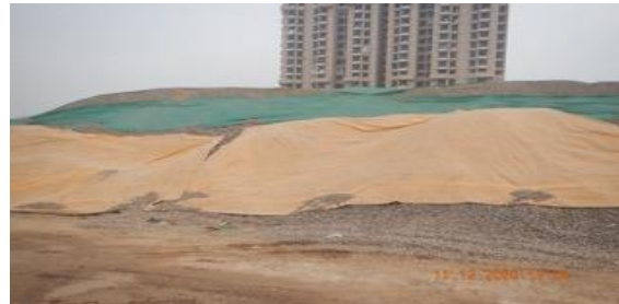
Fig 10 Stockpiles covered with tarpaulin sheets
