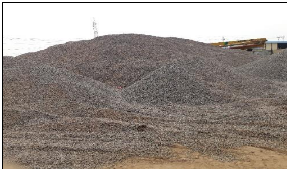
Fig 9 Storage of Coarse Aggregates w/o Dust Suppression Measures
