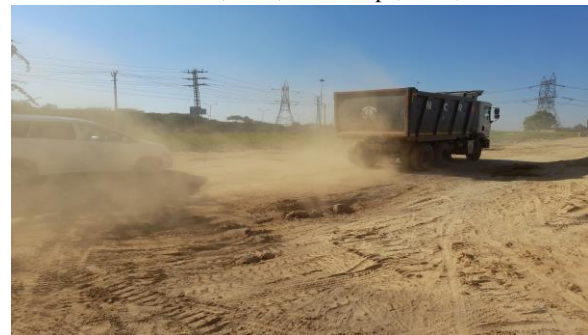
Fig 7 Uncontrolled road dust in haul roads
