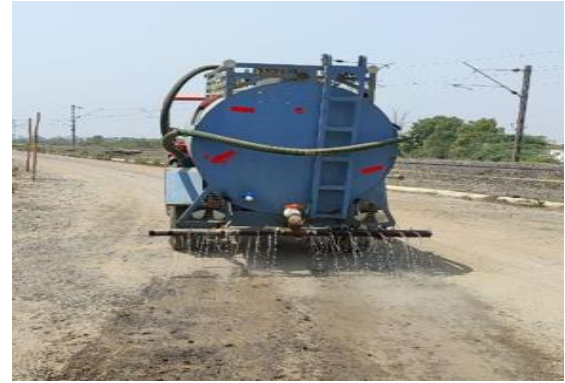
Fig 13 Water Sprinkling arrangement
