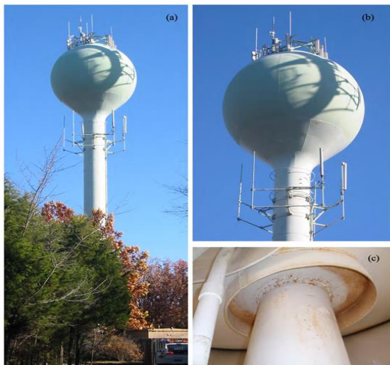
FIG. 9 Exterior view of water tank ( https://www.researchgate.net/profile/KirkGrimmelsman/publication/269198325_Structural_Identification_of_an_Elevated_Water_Tank/links/56c8c7a308ae96cdd06bb78 )
