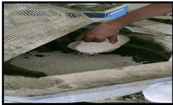
Fig 1: Mixing of EPS beads concrete
