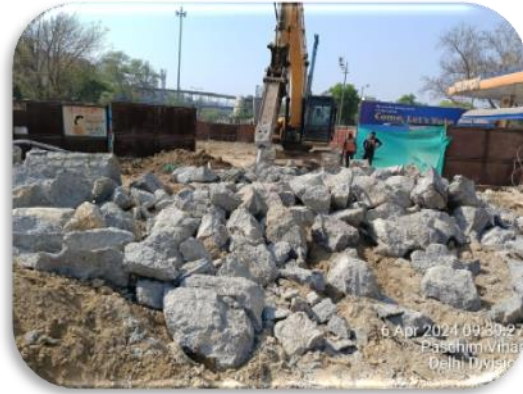
Photo-2 : Construction Machine (Breaker)
