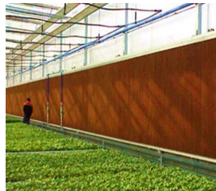
Greenhouse at hot climate with mist, air circulation fan and cooling pad
