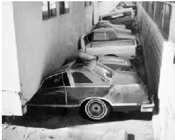
Fig.1.a Soft story collapse, Los Angles, 1994 [5].
