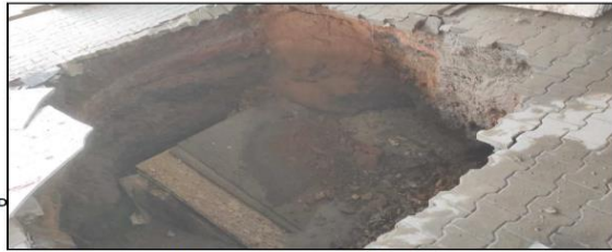
Fig. 15: Showing grouting is under progress
