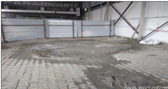
Fig. 17: Showing grouting work at sink hole location
