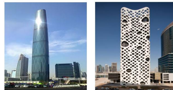
a. Guangzhou Twin Towers b. O-14 Building in Dubai
