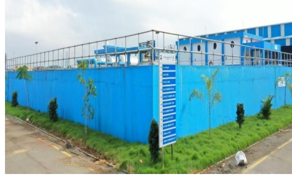
Fig. 5 Treated water storage Tank
