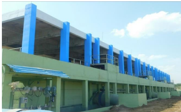
Fig. 2 Rapid Gravity Filters building
