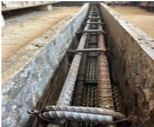
Fig 3 Reinforcement rebar with Mesh
