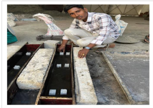
Fig 8.1.2 Casting of Beam
