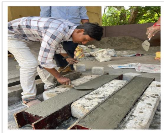
Fig 8.1.4 Casting of Beam
