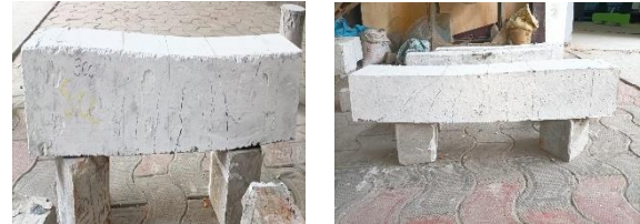
FIG 5 Crack Pattern on Scc & Scgc Beam
