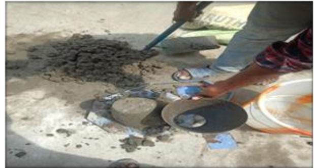
Figure 2 Slump Cone Test
