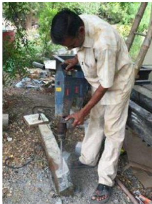
Drilling of Beam specimen
