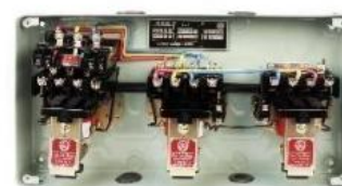
Fig 10. Star Delta Starter
