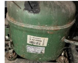
Fig.6:R600a compressor
