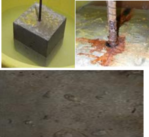
(a) Specimen prior to corrosion (b) Rust deposition at steel concrete interface (c) Outer Concrete Surface Subjected to Spalling
