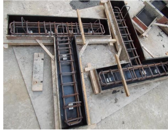
Fig.2 Mould Placed for concrete
