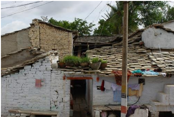
Fig.26. lime stone roof.
