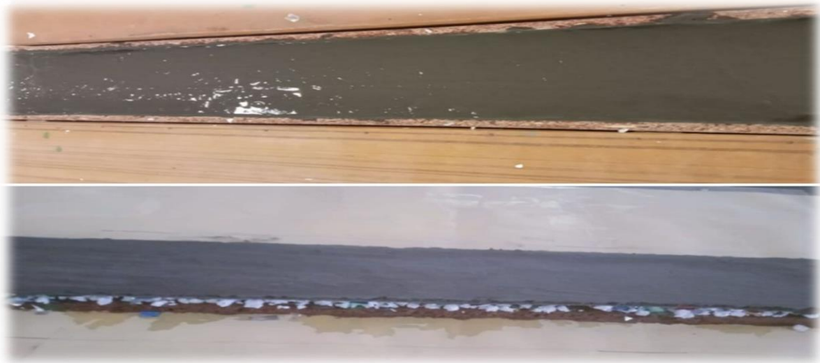
Fig 4- Layer of recycled plastic road surface course
