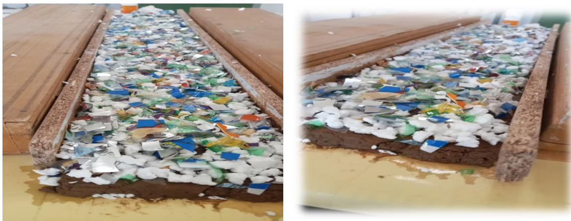
Fig 3- Layer of recycled plastic road base course plastic material
