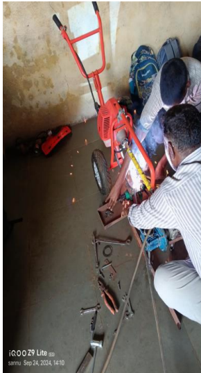
Fig no. 15 Fixing of vibrator
