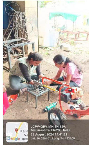
Fig no. 11- Fixing of shaft
