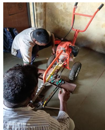
Fig no. 14 Fixing of vibrator
