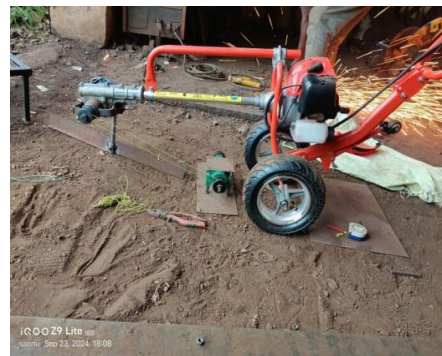
Fig no. 13- Aligning of Vibrator
