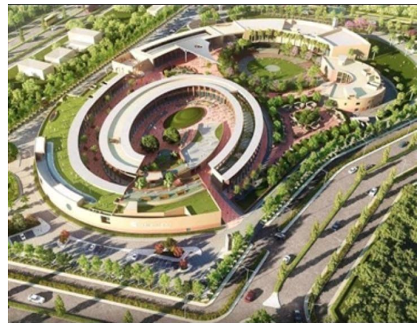
FIGURE 1. 18. Circular buildings in Lucknow
